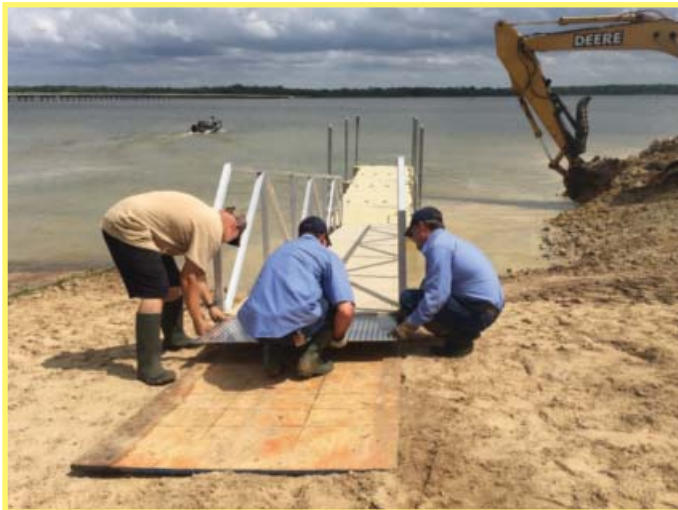
New Floating Pier at the FM515 East Boat Ramp
