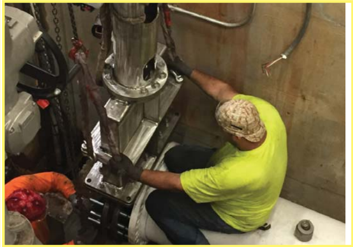
Replacement of 20" Spillway Discharge Valves
