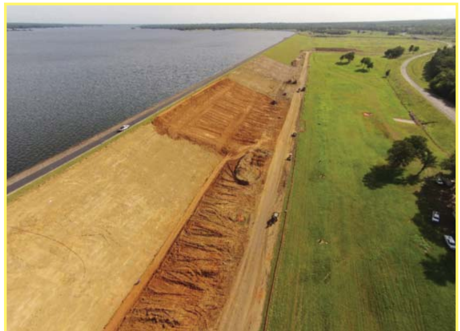
Soil Replacement Project
