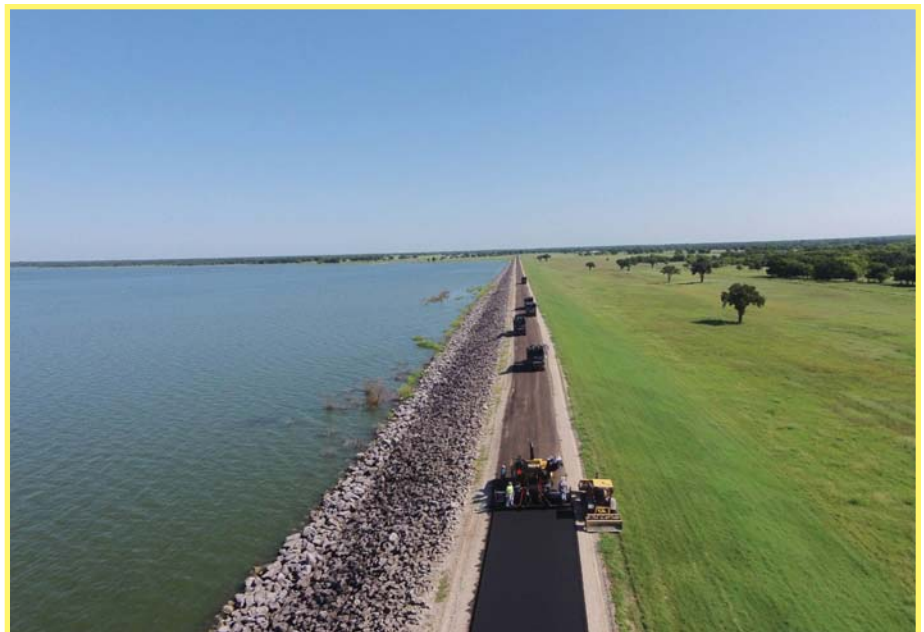
Repaving Road on the Iron Bridge Dam
