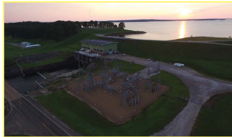
Toledo Bend Dam and Powerhouse
