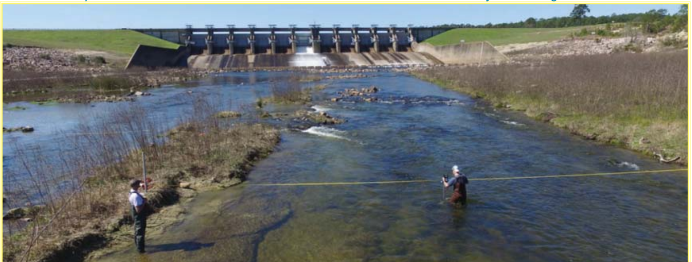
Toledo Bend Spillway Flow Measurement
