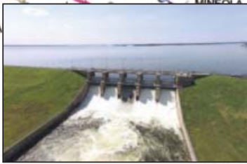
Lake Fork Dam & Reservoir
