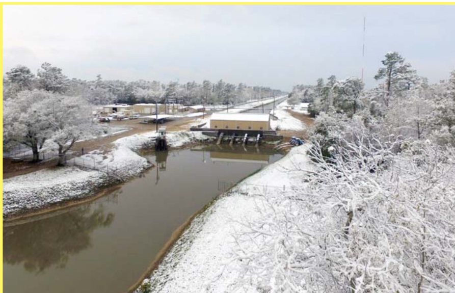
GCD Pump Station
