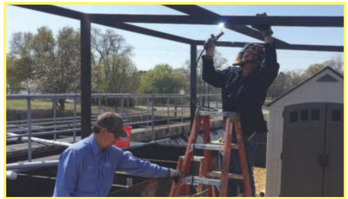
Improvements at the Lake Fork Country Club Estates Wastewater Treatment Facility
