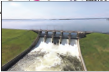
Lake Fork Dam & Reservoir
