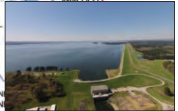
Toledo Bend Dam & Reservoir
