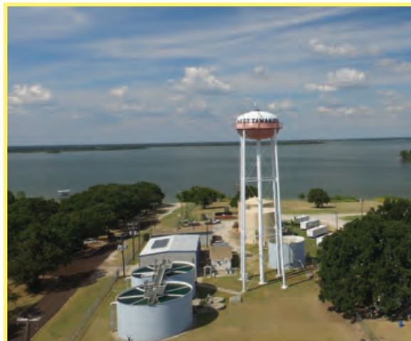
West Tawakoni Water Treatment Facility
