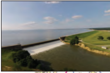
Iron Bridge Dam & Reservoir (Lake Tawakoni)
