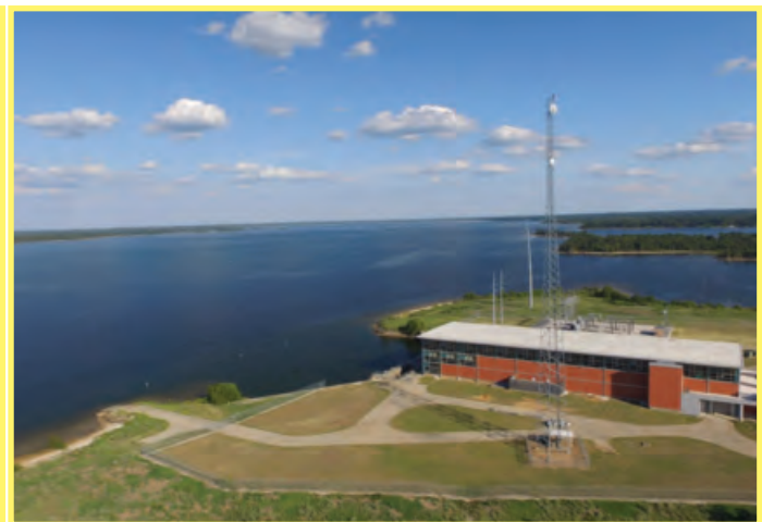
The City of Dallas Raw Water Intake Structure
