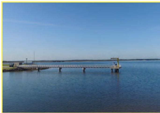
The City of Quitman Raw Water Intake Structure
