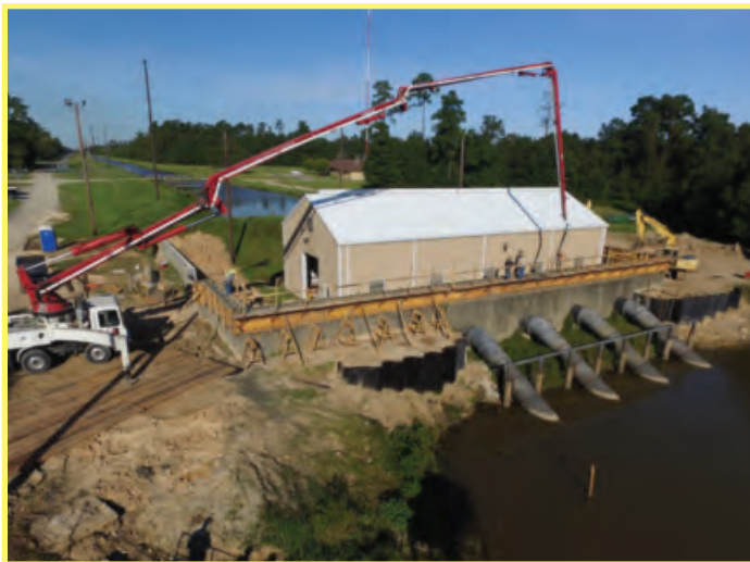
Four-Foot Addition to the Pump Station Flood Wall
