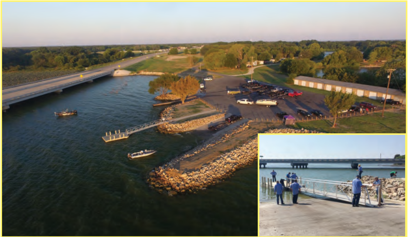
Newly Improved Two-Mile Bridge Boat Ramp Facility
