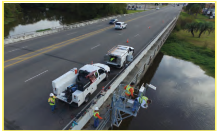
USGS Installing New Gage at Adams Bayou in Orange
