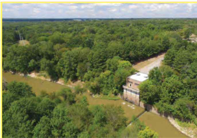
The City of Longview Raw Water Intake Structure
