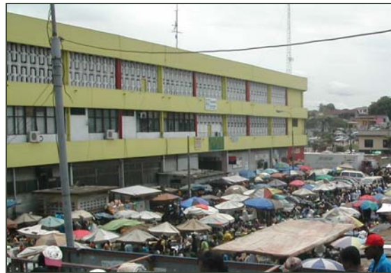
Lack of adequate road space for vehicles
