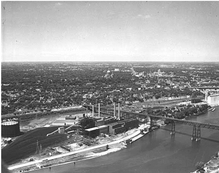
Figure 14. NSP High Bridge Plant (1924), in 1958, looking northeast.
