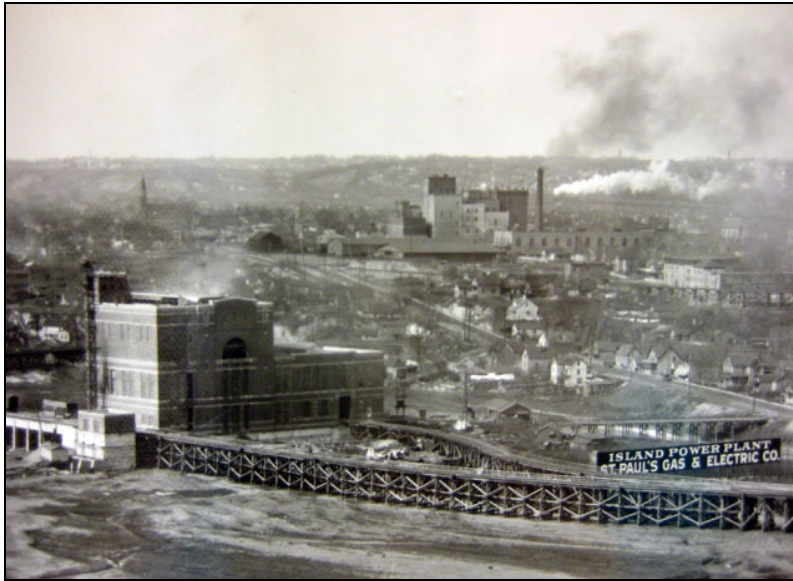
Figure 16. Island Power Plant Station construction, looking northwest, ca. 1924. (NWAA)
