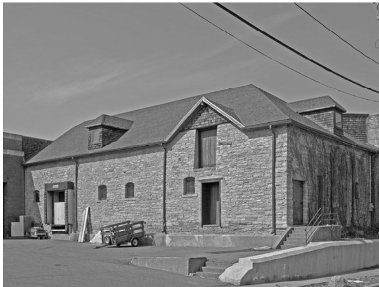
Stahlmann Stable, view from southeast, SBHD11a.2
