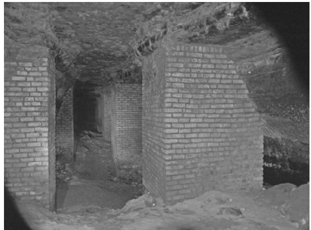
Piers in Schmidt-era cellars, SBHD8.2
