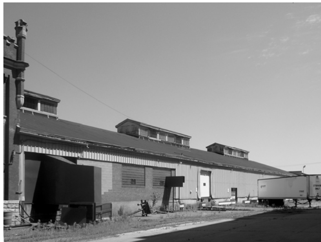
Bottle Warehouse, view from northwest SBHD2b.1 (June 20, 2005)
