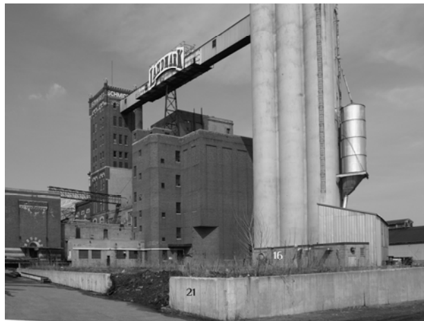
Retaining Wall (21) and Stock House Cellar Entrance (16), view from southwest
