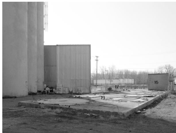
Tank Farm Platform (19), Stock House Cellar Entrance (16), and Cooling Plant Support (17), view from northwest
