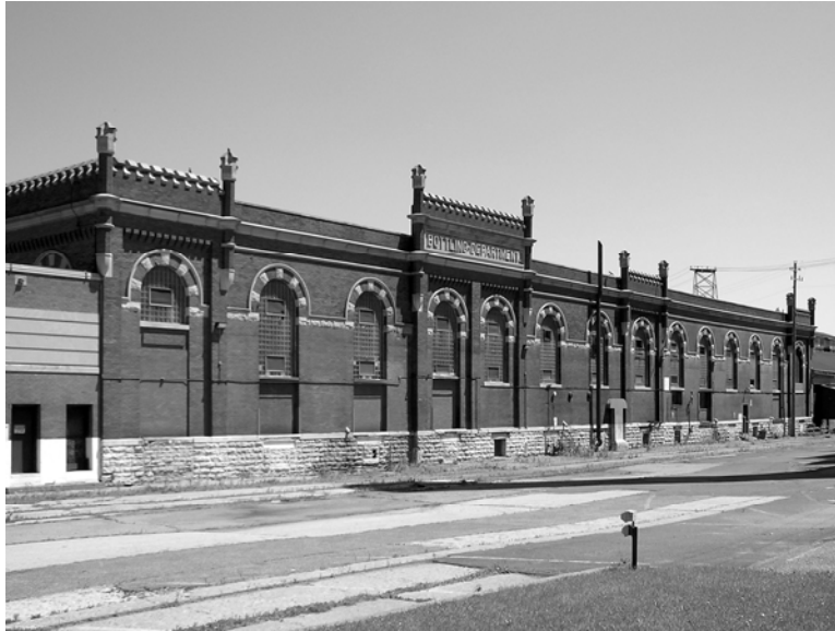
Bottle House, view from northwest, SBHD2a.1 (June 20, 2005)
