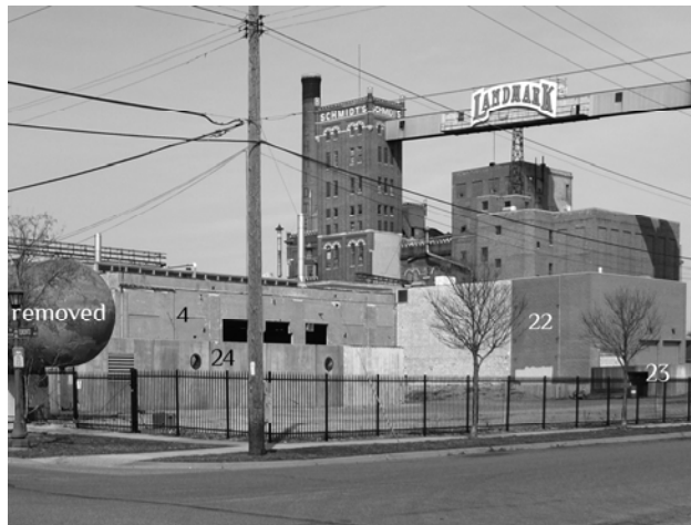
Ethanol Control Room (24), Keg House (4), Ethanol Cooling Plant (22), and Corn Silo Foundation (23), view from southwest
