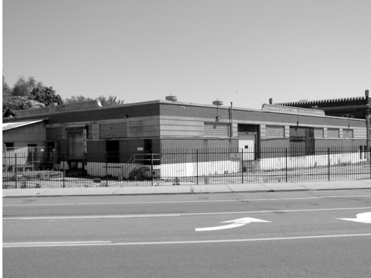
Bottle Shipping House, view from northwest showing covered Truck Unloading Dock and Truck Ramp (noncontributing components) SBHD2c.1 (March 28, 2008)
