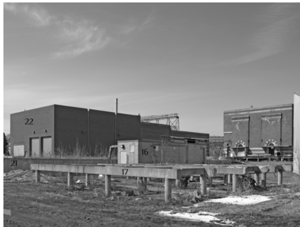
Cooling Plant Supports (17), Stock House Cellar Entrance (16), Retaining Wall (21), and Ethanol Cooling Plant (22), view from southeast
