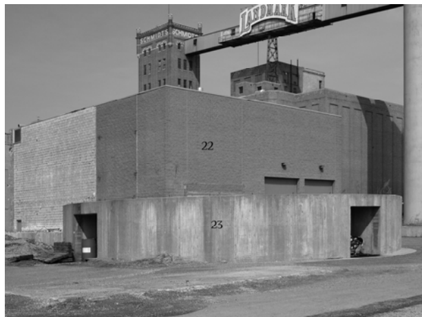
Ethanol Cooling Plant (22) and Foundation of Corn Silo (23), view from southwest
