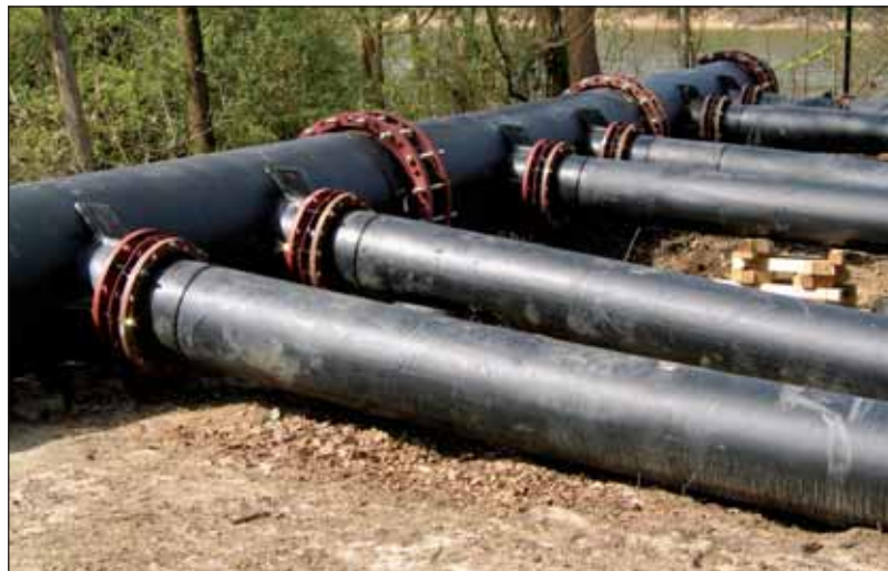
HDPE pipe is ideal for large pump installations requiring high flow rates and long discharge lines
