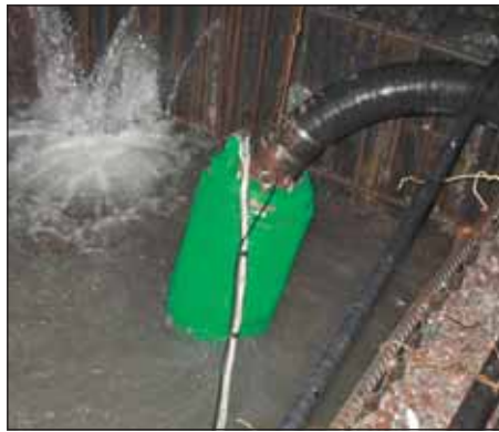
Mody 4" 10 HP Dewatering Pump Operating in a dewatering application.
