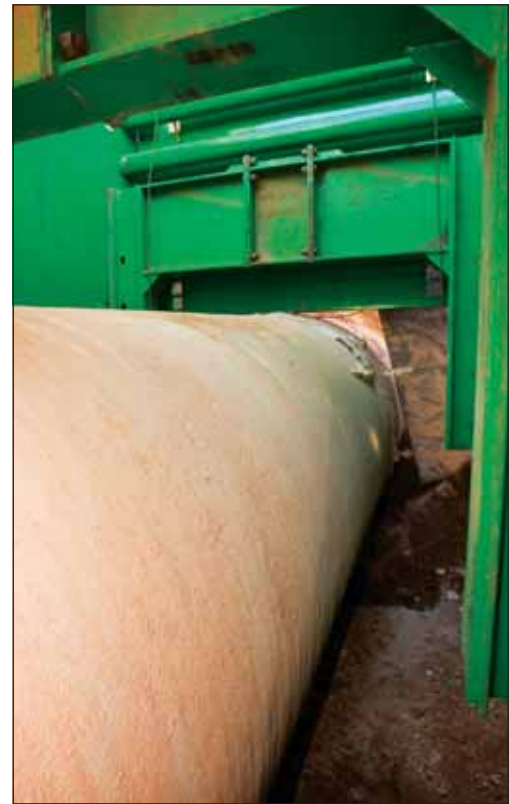
Left: This application required the 76" pipe clearance of a 10' tall trench box. A 10' x 20' 6" wall steel trench box, with an 8' x 20' 6" wall box stacked on top, provided the necessary 18' of protection while reducing weight for easier movement.
