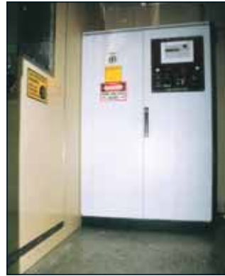
Left: Generators include a digital control panel located in an isolated control room for security and weather protection. Right: Walk-through engine compartment provides convenient access to all major components. Includes a 24V DC battery lighting system
