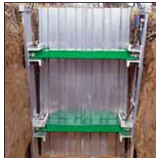
Vertical end shores are available for shoring the end of the trench.
