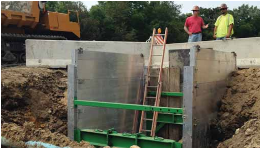
A custom engineered shoring installation on a natural gas transmission line project. Two 8' x 16' 4" wall aluminum trench boxes with 20' steel spreaders were utilized
