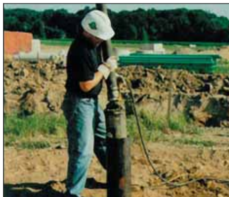
2" Dewatering pump being lowered inside a narrow casing
