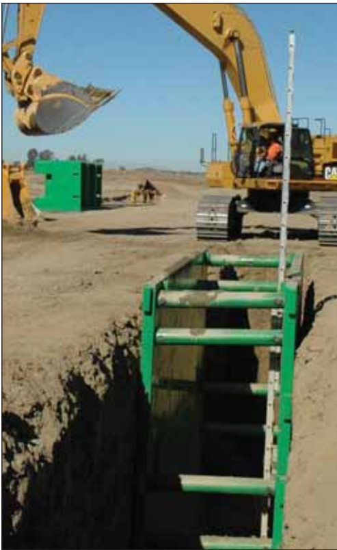
Left: This application required the 76" pipe clearance of a 10' tall trench box. A 10' x 20' 6" wall steel trench box, with an 8' x 20' 6" wall box stacked on top, provided the necessary 18' of protection while reducing weight for easier movement.
