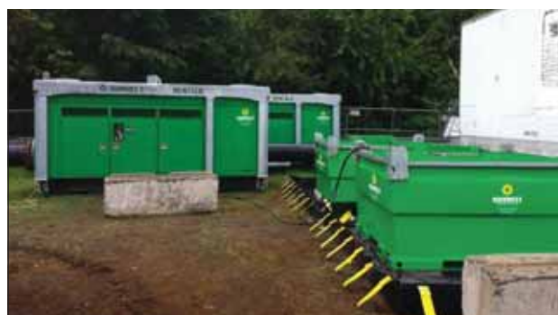
Two containment berms holding auxiliary fuel tanks at a dewatering project in Seattle, WA
