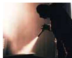
Surface Preparation Protective Coating Application
