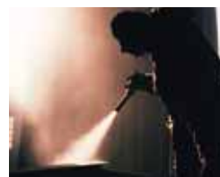
Surface Preparation Protective Coating Application
