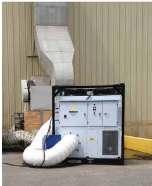
Combined Refrigeration SACP40A-HS 40-ton Industrial Air Conditioner
