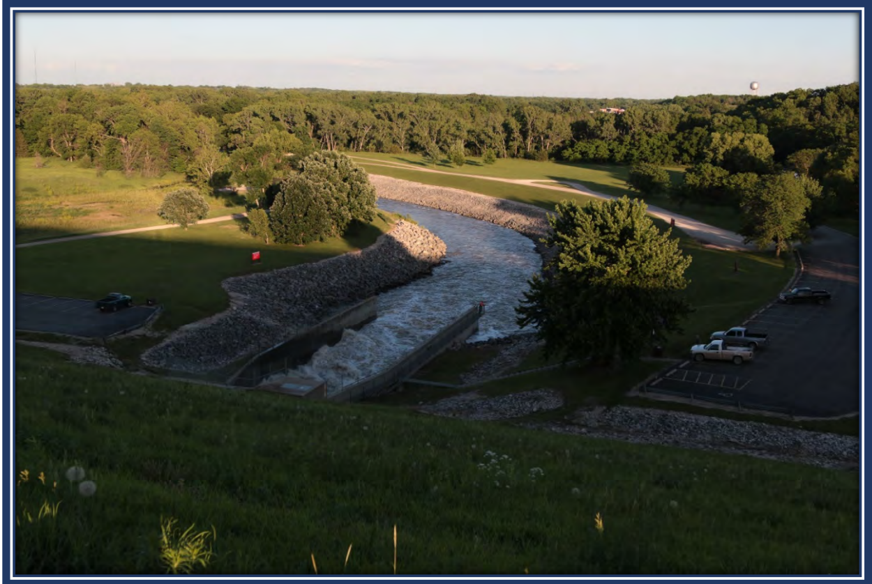
Photo 5-1 Outlet Channel day use parks, Council Grove Lake (Source: USACE)
