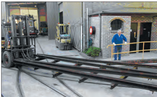
A section of completed pointwork is moved from the top yard.
