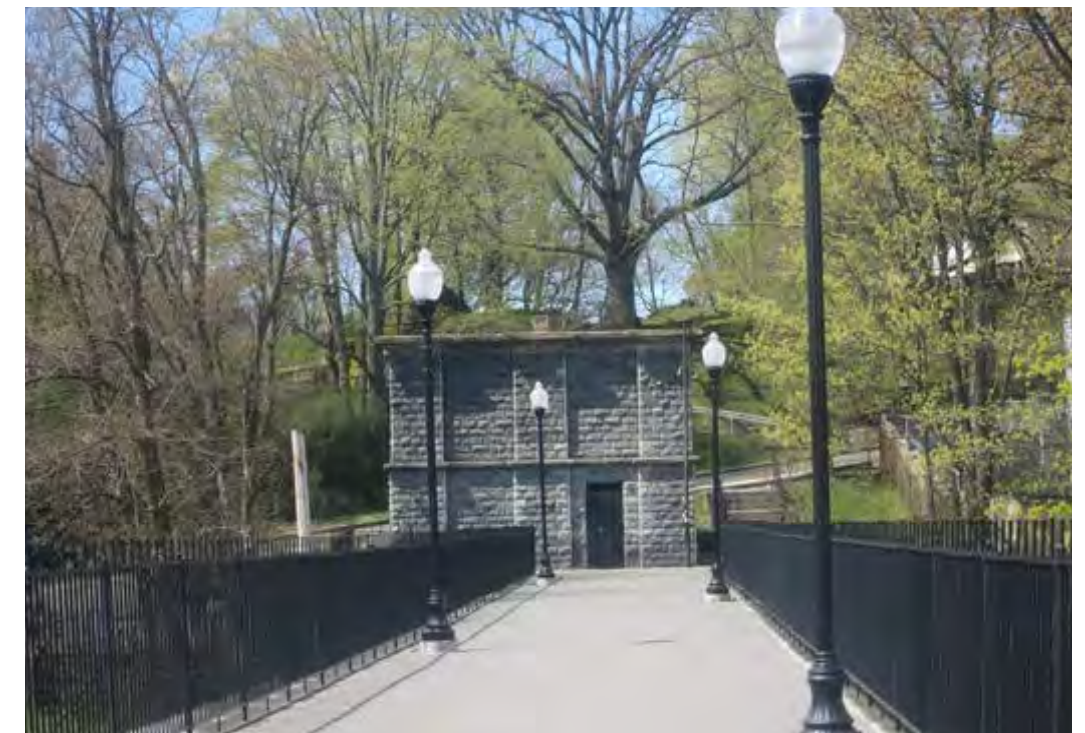
Old Croton Aqueduct structure
