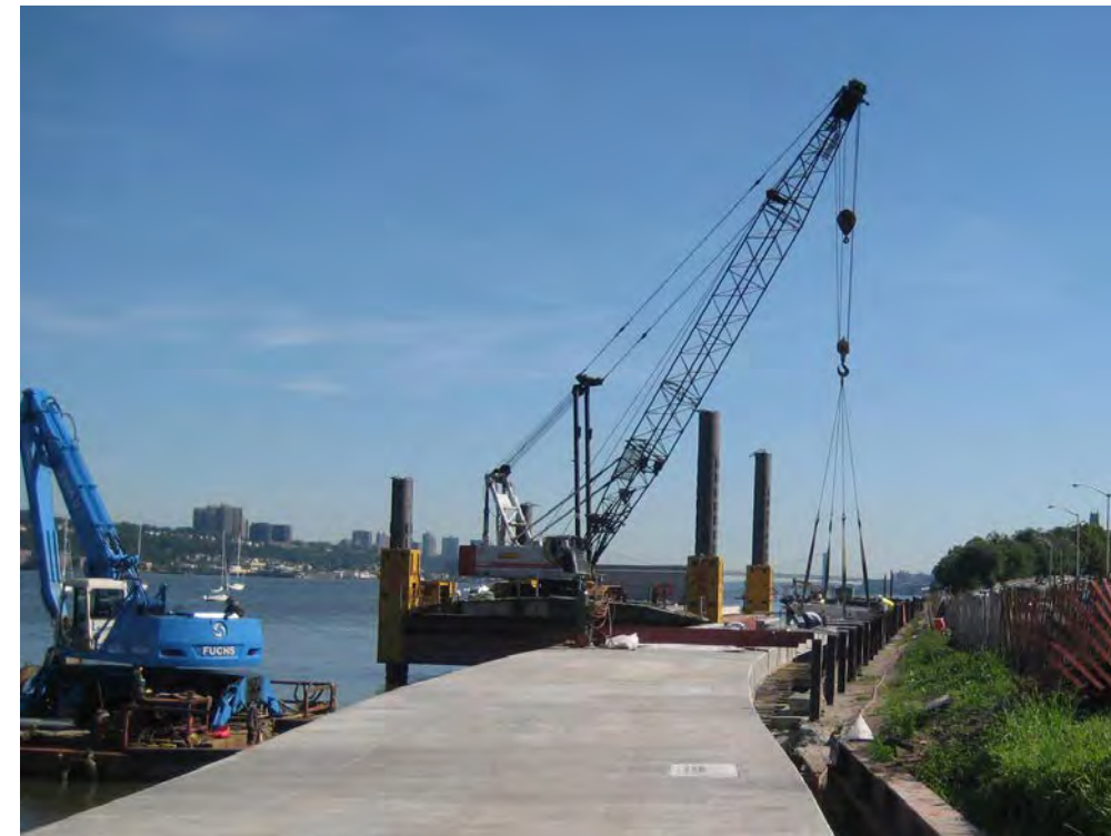
Typical Working Barge with Crane
