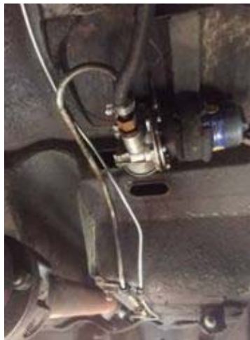
Inlet/Outlet at stock fuel pump (Note: the rubber portion of the line is INCORRECT. The line was steel all the way to the inlet valve on pump.)
