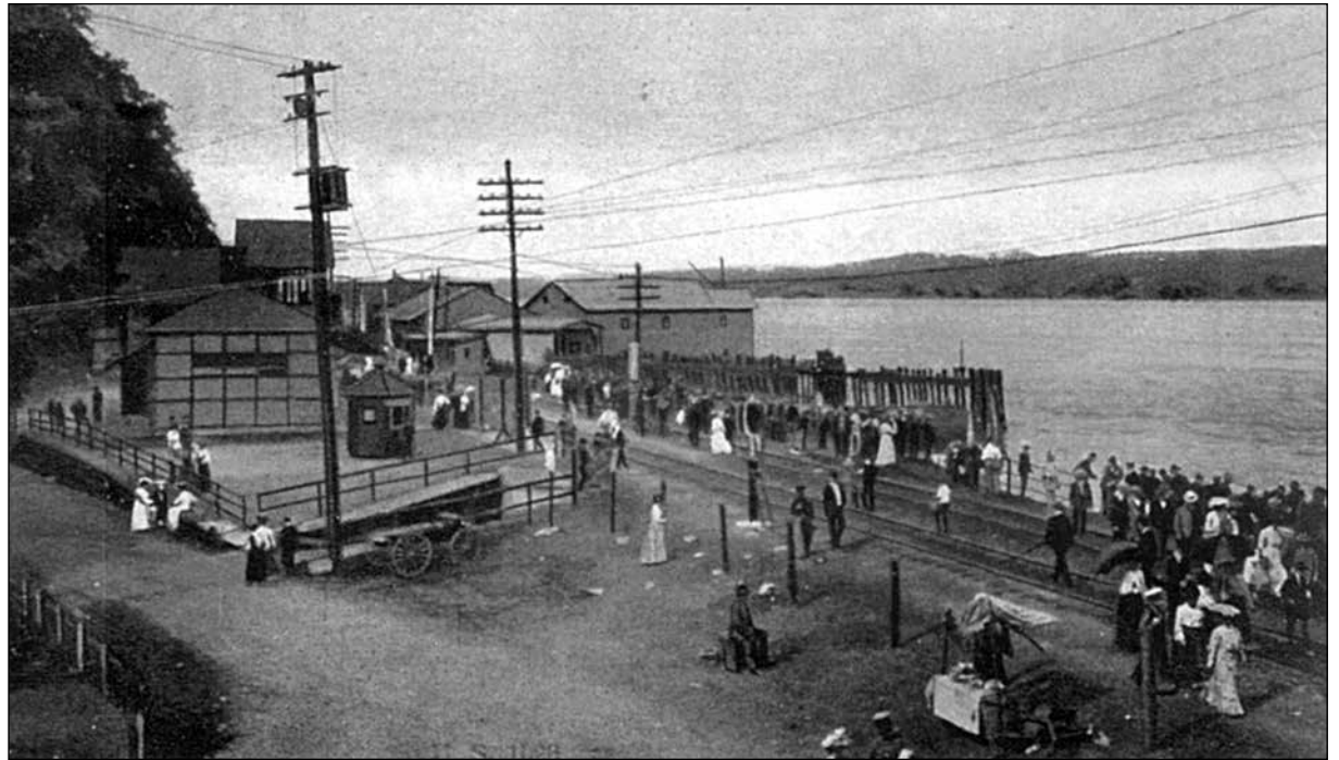
Seen here is a northbound view of the West Shore Railroad Depot complex in Highland, which illustrates the popularity and multiple functions of this hub. The piles in the Hudson River show where the ferry landing was. The ferry crossed the river to Poughkeepsie where passengers could transfer to the day liners that ran from Albany to New York City. This ferry service ran until 1941, when World War II fuel scarcity fully impacted the United States.
