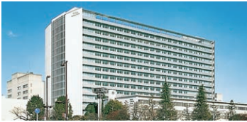
Head Office Technical Center (Toyota City, Aichi Prefecture, Japan)
