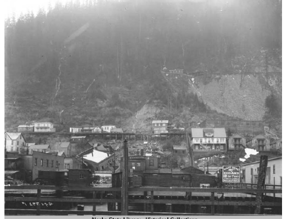
Photo 38. Gastineau Avenue Landslide in 1920s Juneau. Alaska State Library Historical Collections
