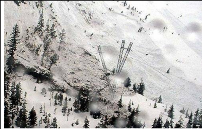
Photo 30. Courtesy Of Mike Laudert / Alaska Electric Light & Power Co.
