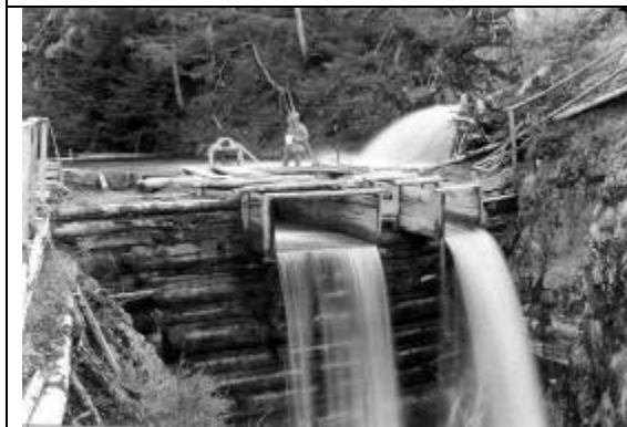
Photo 35. Treadwell Ditch 1905 Alaska State Library Digital Archives
