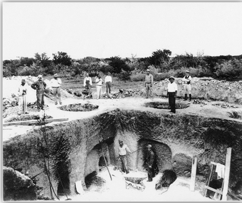
Figure 20. Caliche pit, ca. 1934 during mining for the McAllen storm sewer project. Pit later filled with water and is the site of the lake on Tom and Cristina Eubanks' property-Location 2. Photo courtesy of Carroll Norquest.
