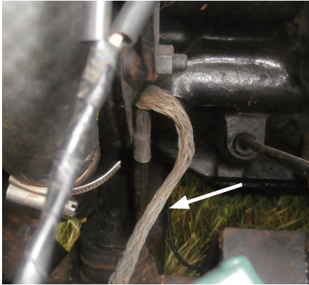
12.2: Often overlooked, the earth strap is a vital bit of the TR's electrics.
