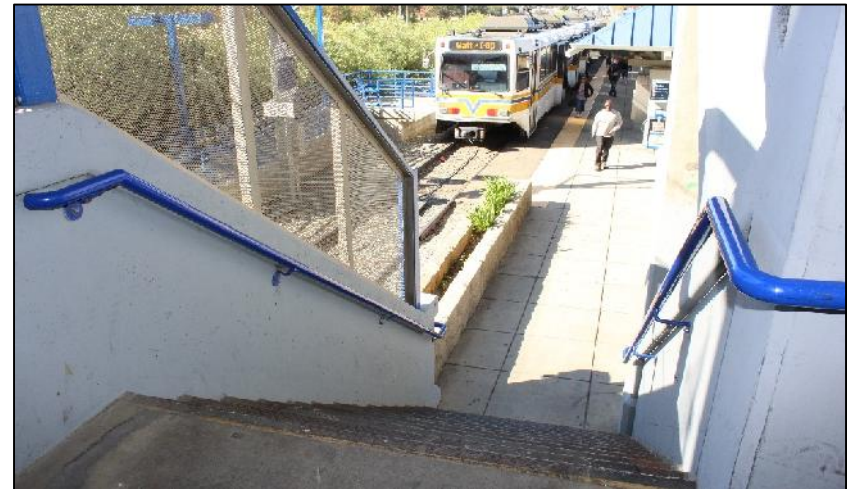
Riders recommended redesigning the stairs and replacing the elevators to improve transfers.
