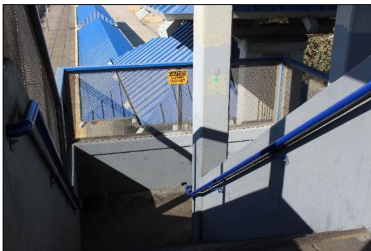
Shadows, sharp corners, and concrete columns create hiding spaces and contribute to safety concerns.
