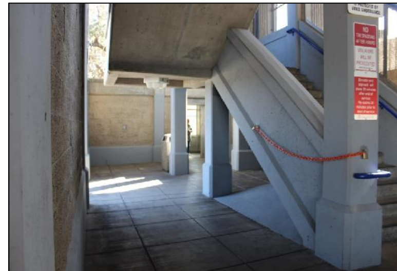
Columns and the staircase create multiple hiding spaces and block visibility of the elevator.
