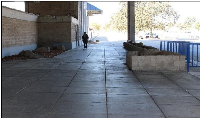
Riders transferring between the northbound bus stop and light rail feel unsafe walking under the overpass area.
