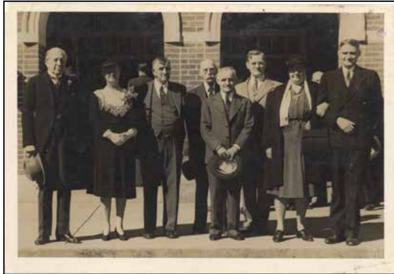
Left: Dedication of New Deal buildings on campus.
