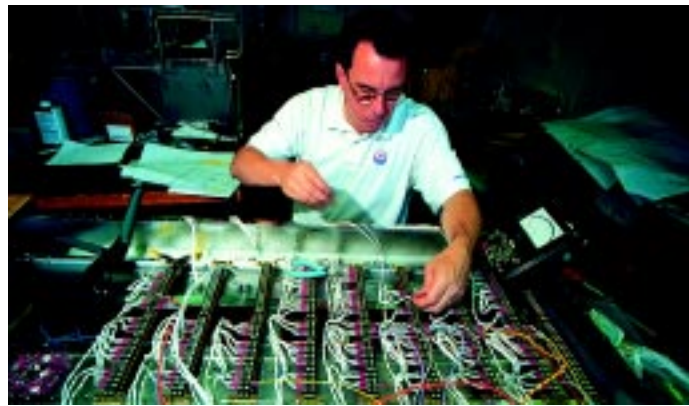
Martin Bowen wires a junction box for LEO-15, the Long-Term Ecosystem Observatory installed in 15 meters of water off the coast of New Jersey in August 1996.
