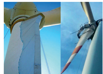
Installing the EvoFlap
