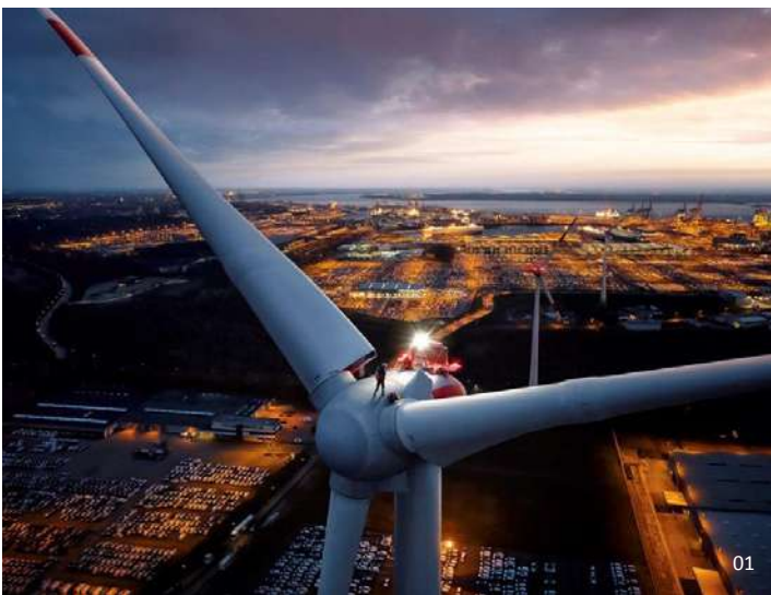
01 | Breathtaking view: This wind turbine has a hub height of 149 meters.
