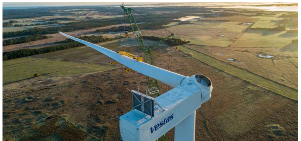
The prototype of the Vestas V162-6.0 MW was erected at the Osterild test site in 2020. Photo: Vestas
