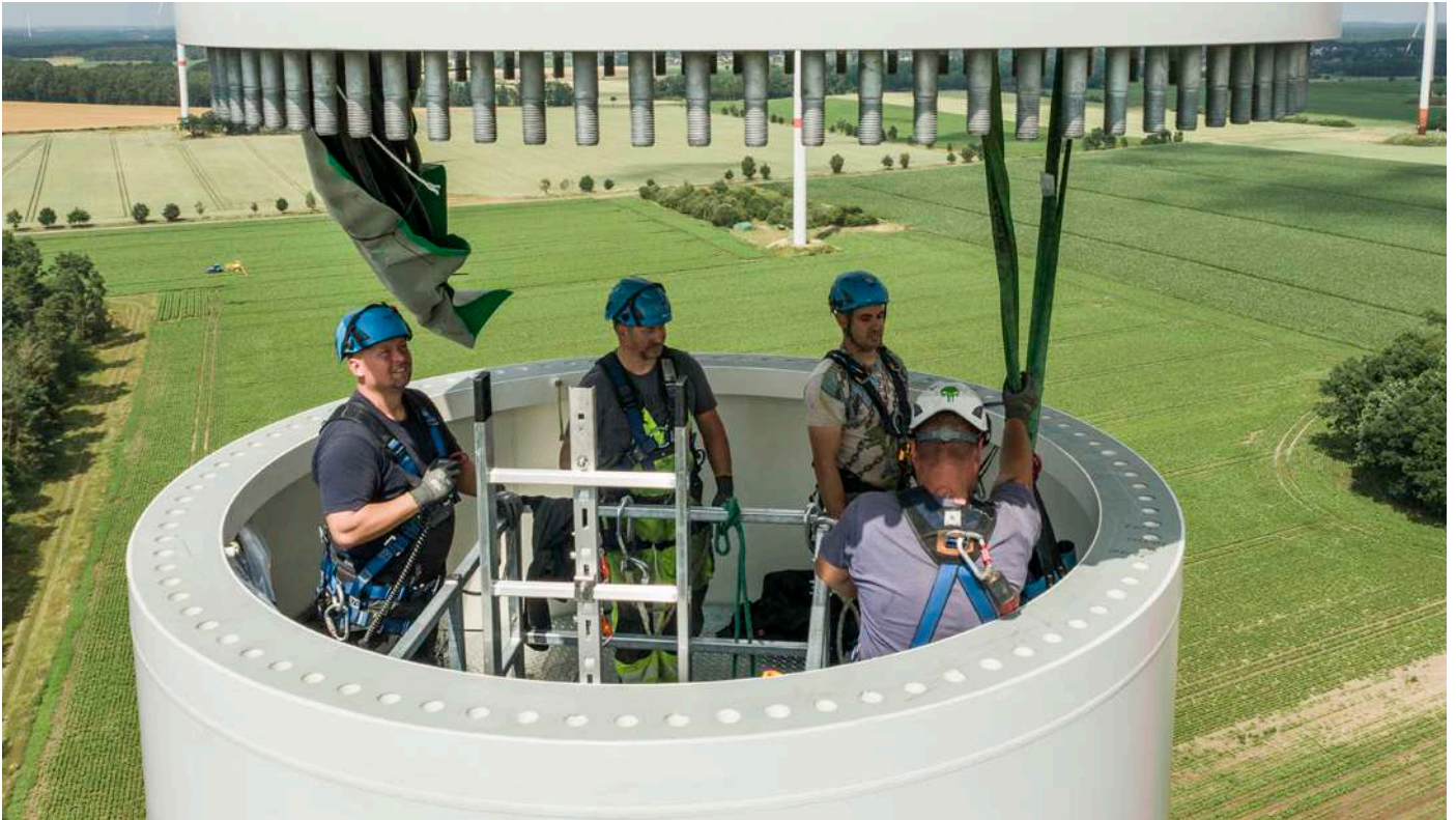
Erecting a Vensys 136, 3.5 MW, hub height 161.2 m. Photo: Ulrich Mertens
