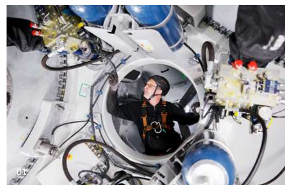
01 | Wind Turbine Technician from enercity Erneuerbare GmbH in a hub of a vestas turbine.
