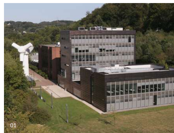
01 | Training Center of KWS Energy Knowledge eG 02 | WPI Training Tower
