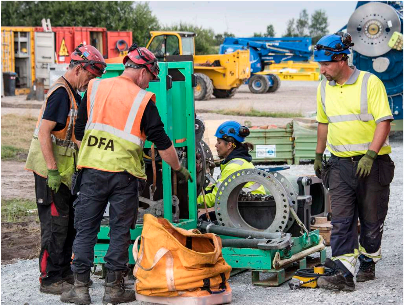
Prototype 1 of the N163/5.X at the test site of Janneby citizens' wind farm. Fitting the hydraulic unit that will correctly position the hub when fitting the rotor blades. Photo: Ulrich Mertens
