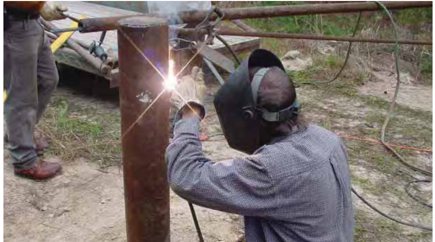
Welding up a new gate post on a WMA.
