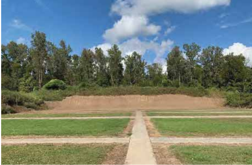
Completed lead reclamation on Sherburne rifle range.
