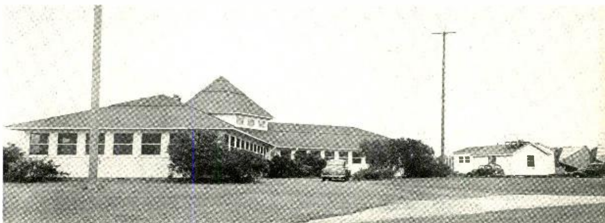
The main building at Holmdel has a central foyer from which radiate two wings housing laboratories and offices, and a third wing for shops and services.
