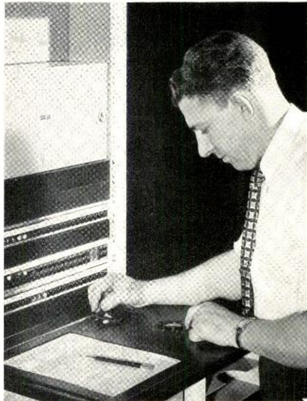
Fig. 2—Maintenance man dials unattended repeater station which responds by lighting lamps under log sheet.
