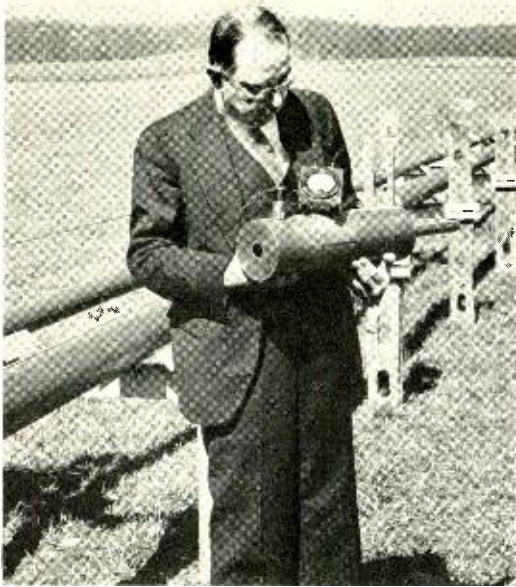
Stretching a quarter-mile from the Roberts House are Holmdel's first two wave-guides.
