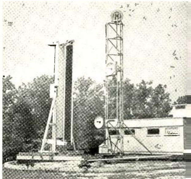
Mounted on a turntable atop Crawford's Hill at Holmdel, this microwave set can be pointed at various objectives—some of them reflectors which allow the transmitting and receiving ends of the path to be operated in the same room.
