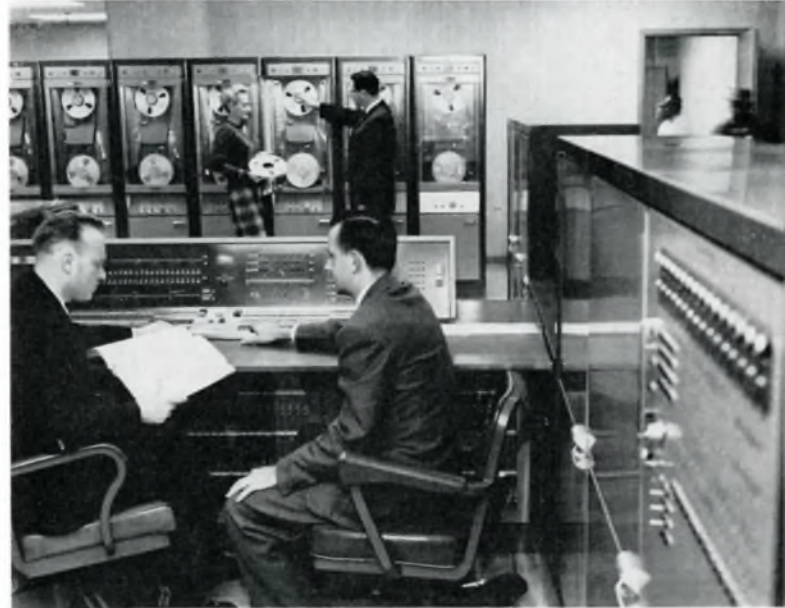
A test program is prepared at the computer operator's console of the new Philco electronic data processing system recently delivered to the Data Processing Center in Plant 2 by Don Bonsall (right), operations supervisor, and Graham Cairns, operator. In the background James Maguire, manager of the Data Processing Center, changes a tape reel on the magnetic tape transport assisted by Myrtle Kemmerer.
