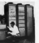
The PSI Auto-Sorter tests for as many as 8 different diode types simultaneously at a rate as high as 8,000 diodes per hour
