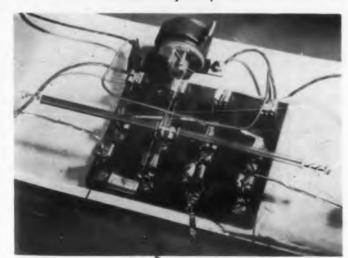
A succession of discs placed along the length of a brass rod has greatly increased the delaying power of this torsional delay line. The signal, which is fed into the line by a torsional transducer, is delayed as much as 114 usec per cm by the difference in diameter between the discs and rod.
