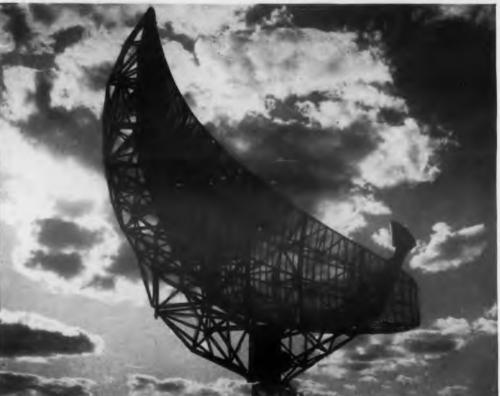
**EXTENDING THE RANGE** of radar is a constant challenge to Raytheon engineers. This 40-foot high-gain L-band antenna was designed to increase the range of existing radar and for use with new radar under development.
