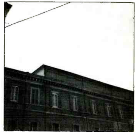
This building which is adjacent to the Poste E Telecomunicazioni building also has antennas on the roof. Photo courtesy of R. C. Watts, KY.
