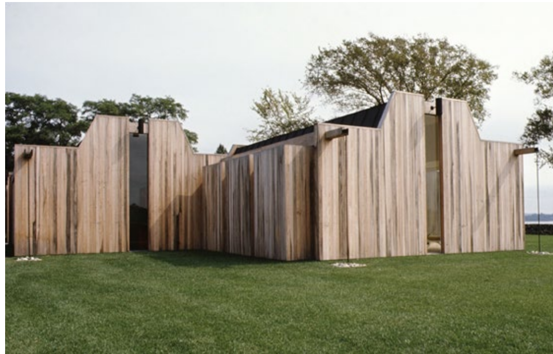
The exterior of Hugh Newell Jacobsen's Pavilion House, also known as the Millet House, located in Bristol, Rhode Island
