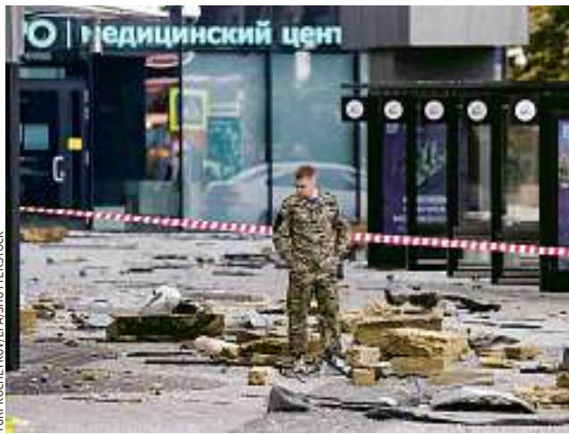
Inspecting debris at the site of a damaged building in Moscow.
