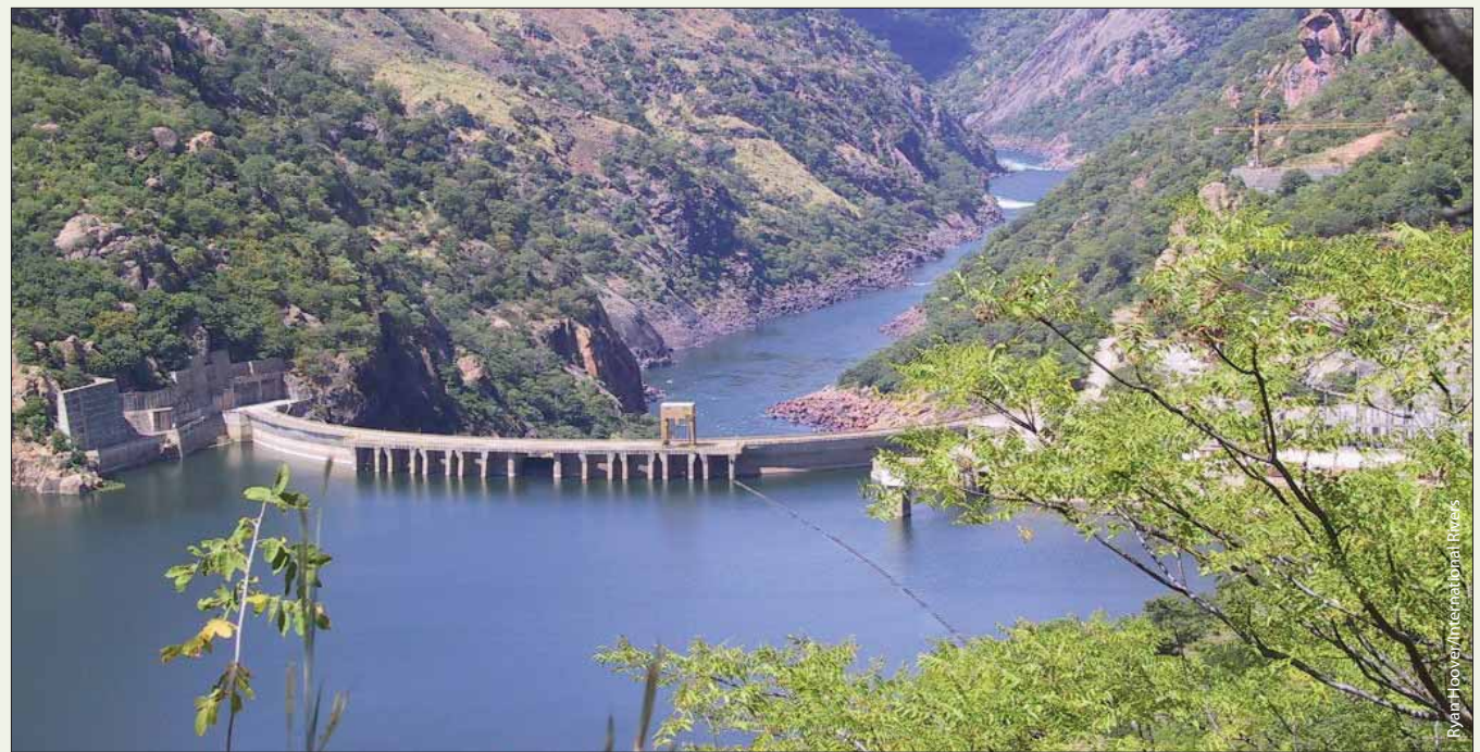
Cahora Bassa Dam in western Mozambique
