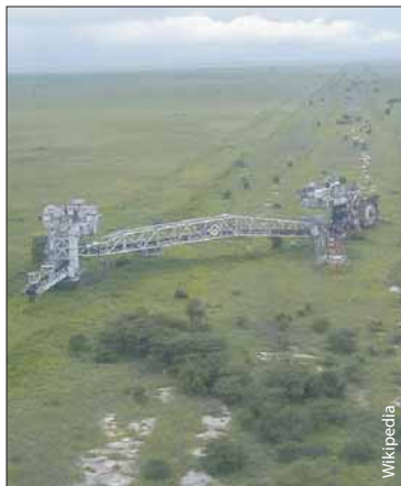
Construction of the canal ended in 1983 and the digger has remained here since
