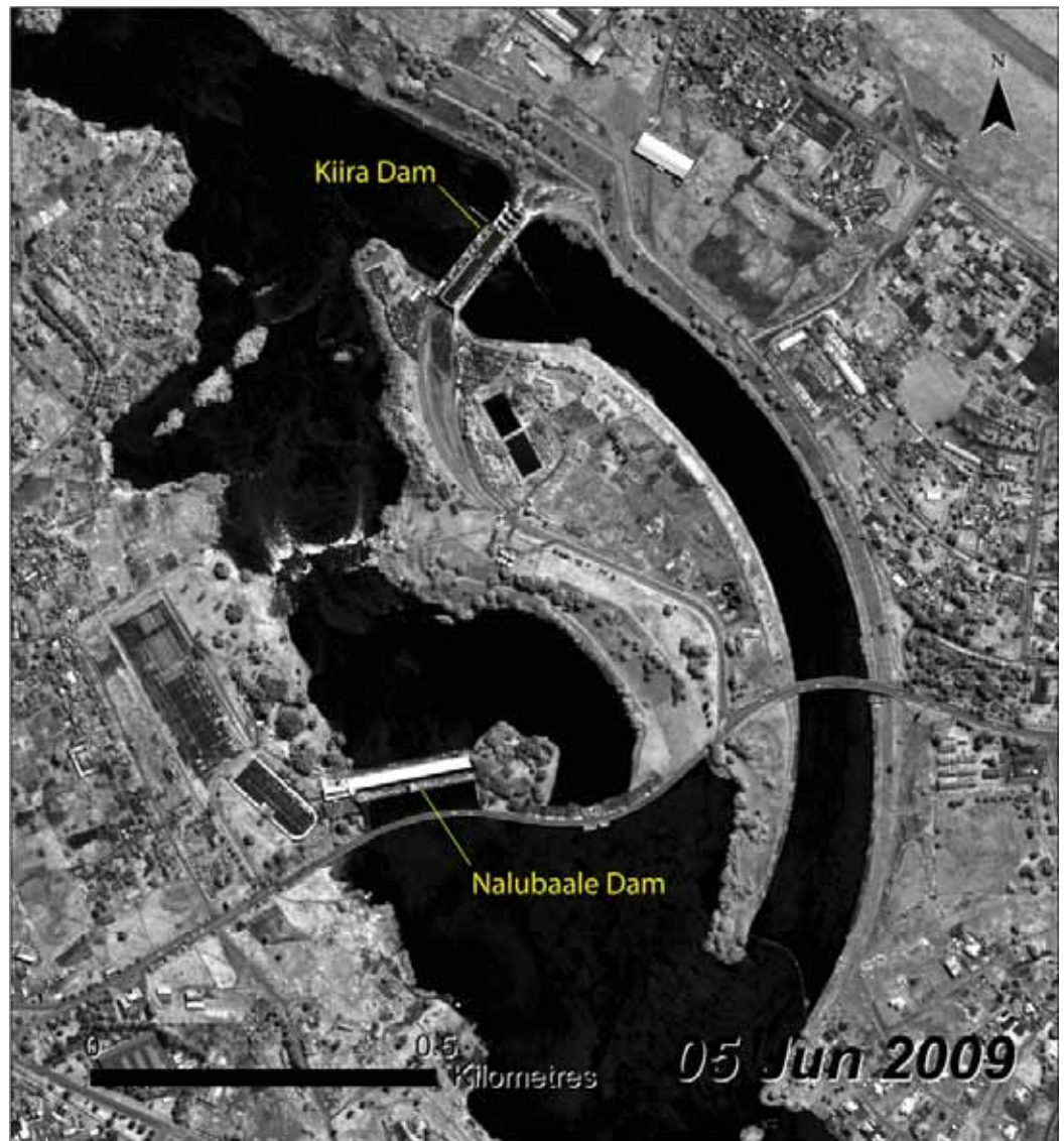
Figure 2.8.7: Location of the Nalubaale and Kiira dams
