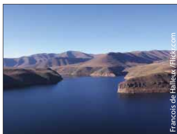
The Katse dam reservoir
