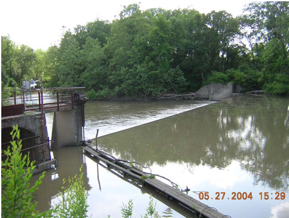
Water Plant Intake
