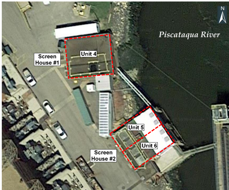
Figure 2. Aerial view of Schiller Station’s Units 4 in Screen House #1 and Units 5 and 6 in Screen House #2.
